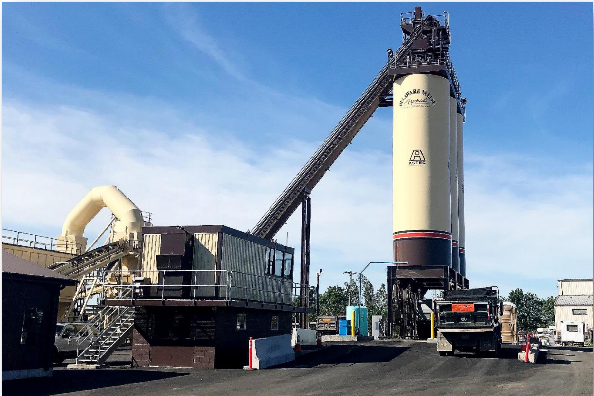
The three 300-ton Astec storage silos bearing the official DVA logo.
