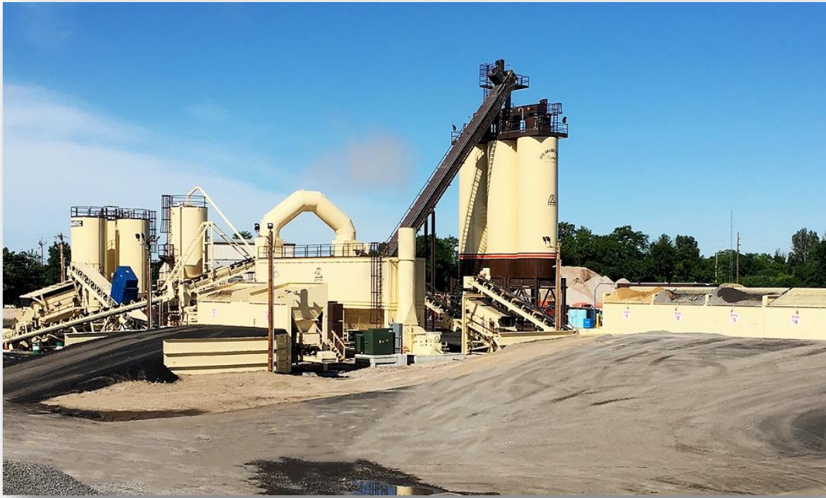
Landscape view of our brand-new facility, including the storage silos, on-site laboratory and multiple material bins. The official logo of Delaware Valley Asphalt.
